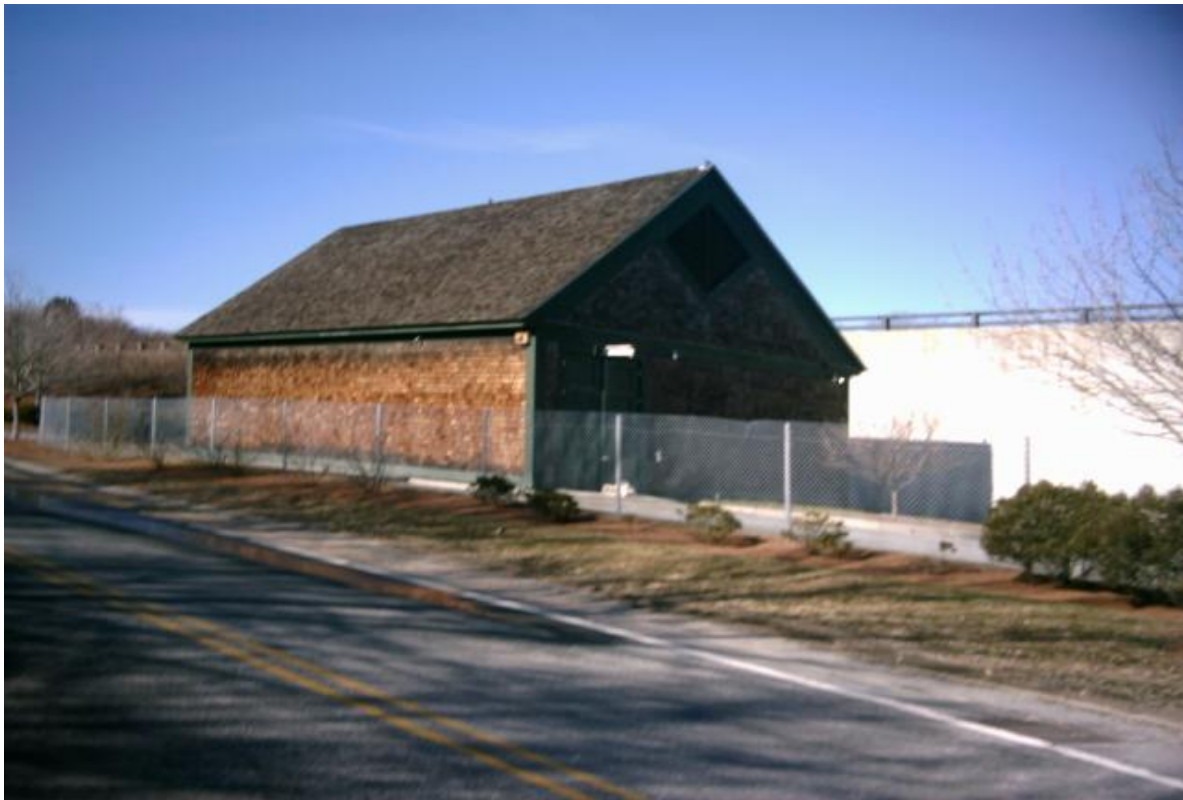
Pump House Building
