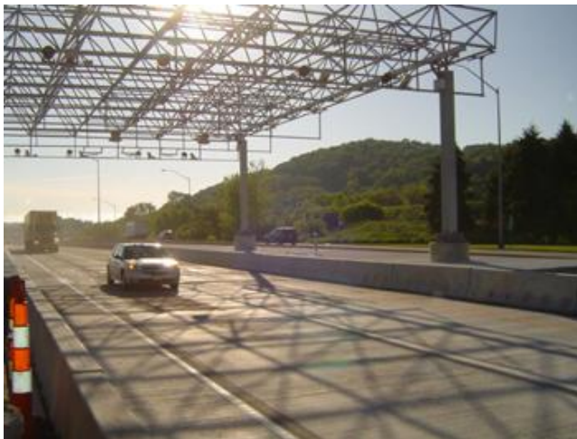
Figure 2: I-78 Express E-ZPass Toll Plaza (DRJTBC website)
